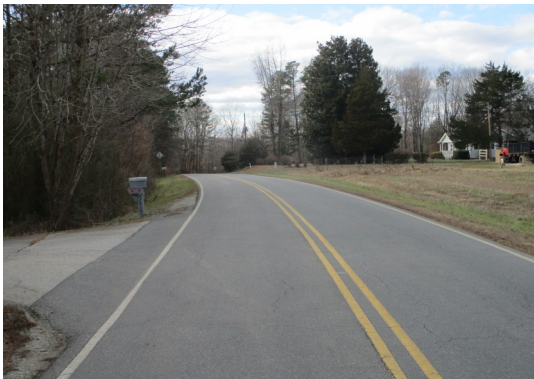
Picture 5: Request location on left as seen looking along Beckerdite Rd.
