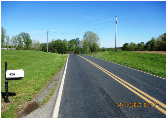
Picture 5: Request location on left as seen looking toward US Hwy 64 E.
